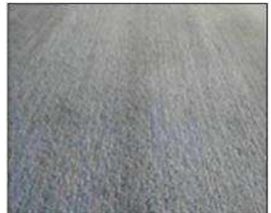
Concrete with K 100 ® -ULTRA after abrasion test
