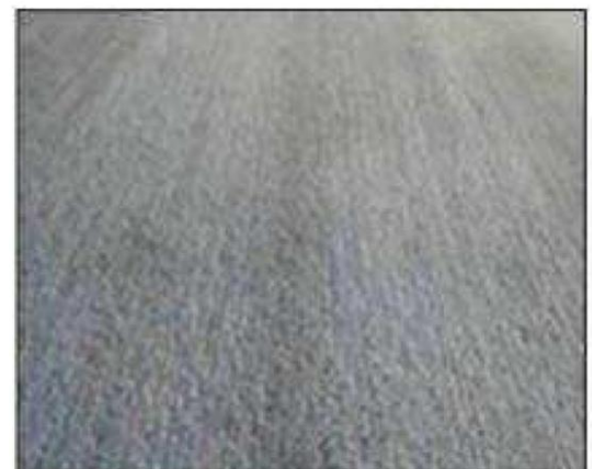
Concrete with K 100 ® -ULTRA after abrasion test
